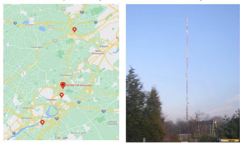
At 988 feet, this tower near the Quakerbridge Mall in Lawrence Township (I-295 at US Route 1) is one of the tallest structures in New Jersey. Mounted on the tower, located at (40.30551, -74.68397) are antennas for New Jersey 101.5 WKXW, Princeton 103.3 WPRB, New Jersey Network 88.1 WNJT, N2RE/R 146.46 MHz FM (David Sarnoff Radio Club Repeater), and others.
